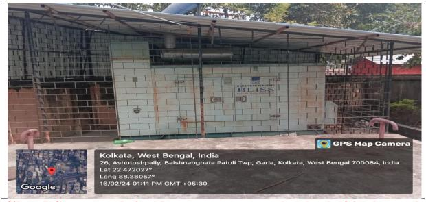
Silent DG sets are designed to generate a very low level of background noise, just as their name suggests. Their structures are constructed to eliminate virtually all noise and vibrations due to careful design. Because of this, they are not harmful to the environment and are ideally suited for use in residential areas.
